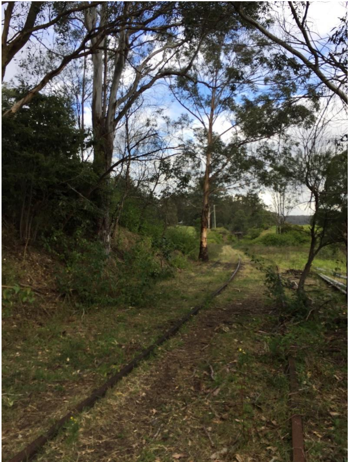
Photograph 4-1 Cleared railway track within the proposal site with fringing vegetation
